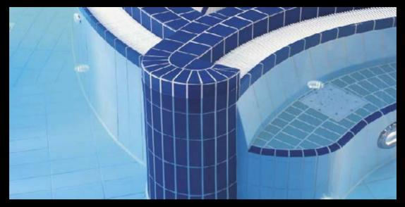
The design of the bench in the Ocean Wave at Norddeich is based on conic cuts. It is impressive because of its high technical quality.
